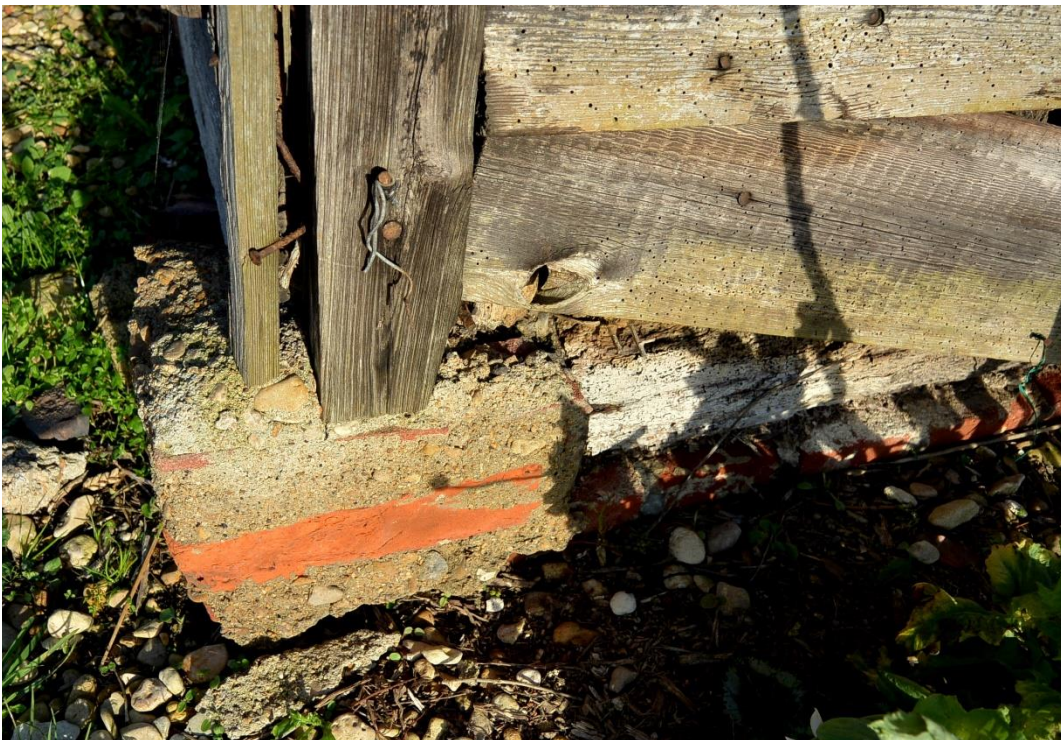
Footings of the front face of the shed and [above]the entrance doorstep
