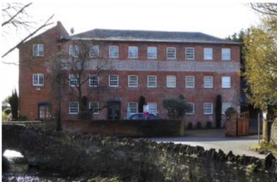
Dandridge's Mill in East Hanney.
