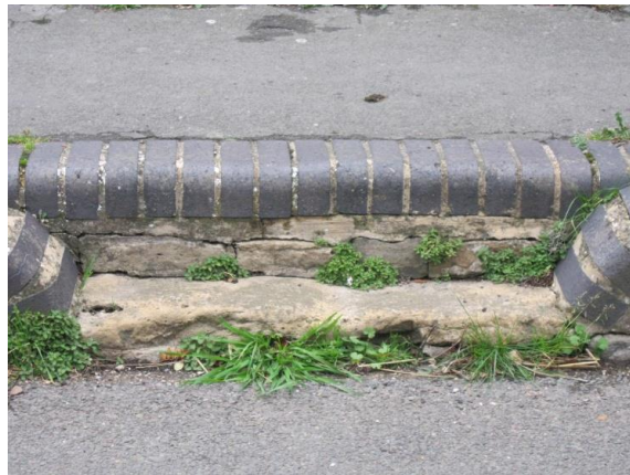
Fig 23 Pavement foundation - Main St. W.H.
