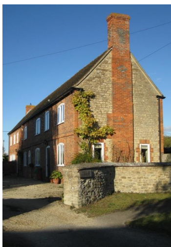
Fig 12 & 13 Use of stone in gable end walls in West and East Hanney, both also using blue and red brick construction
