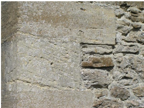
Figs 20 and 21 Ashlars on church tower - the detail on the right shows approx 10" of stone
