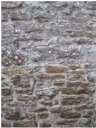
Fig 18 Change of stone in north wall
