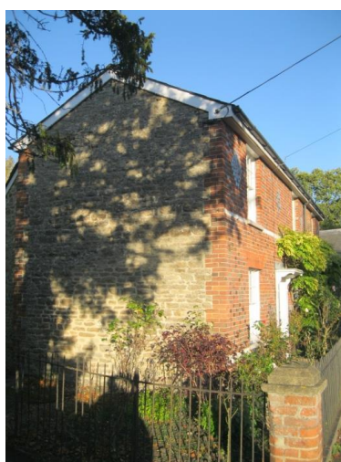
Fig 12 & 13 Use of stone in gable end walls in West and East Hanney, both also using blue and red brick construction
