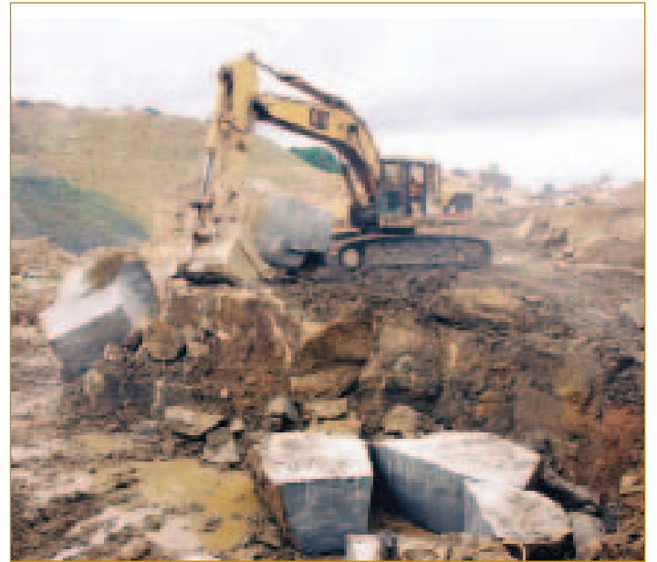
Above and right: Blockstone extraction at Appleton Quarry, using traditional 'plug & feather' techniques to split the stone and mechanical excavators to lift the blocks:
