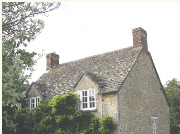
Stonesfield: slate roof with oolitic limestone walls
