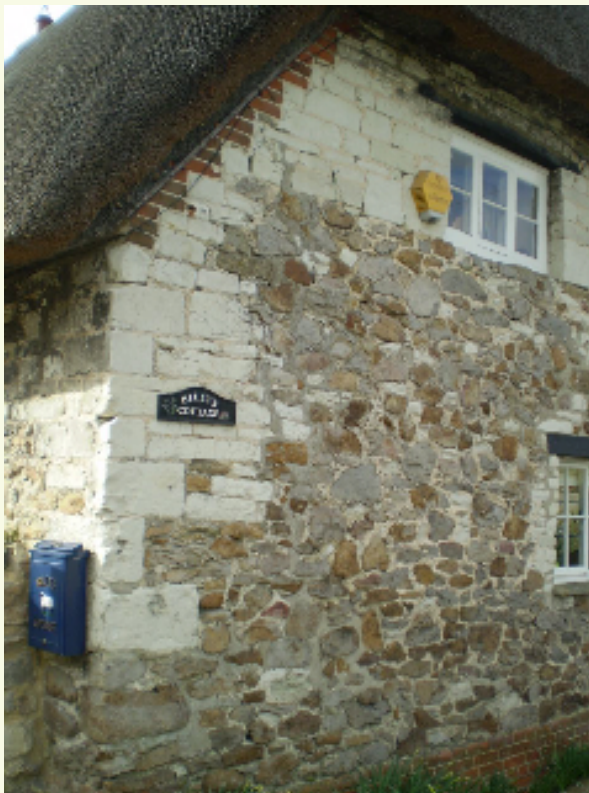
Rough sarsen stonework, with quoins and additions of chalk block, Ashbury
