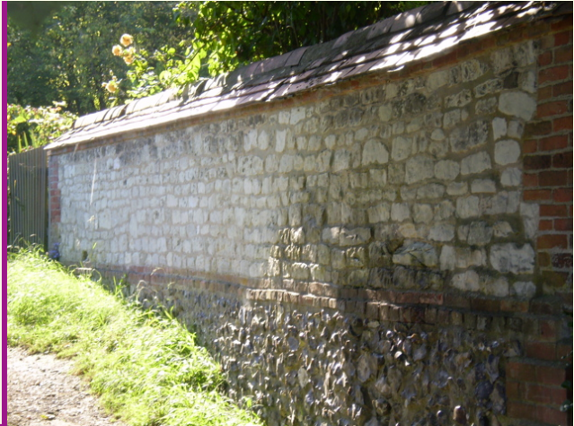
Chalk clunch boundary wall, with protective tile capping and flint base. Blewbury
