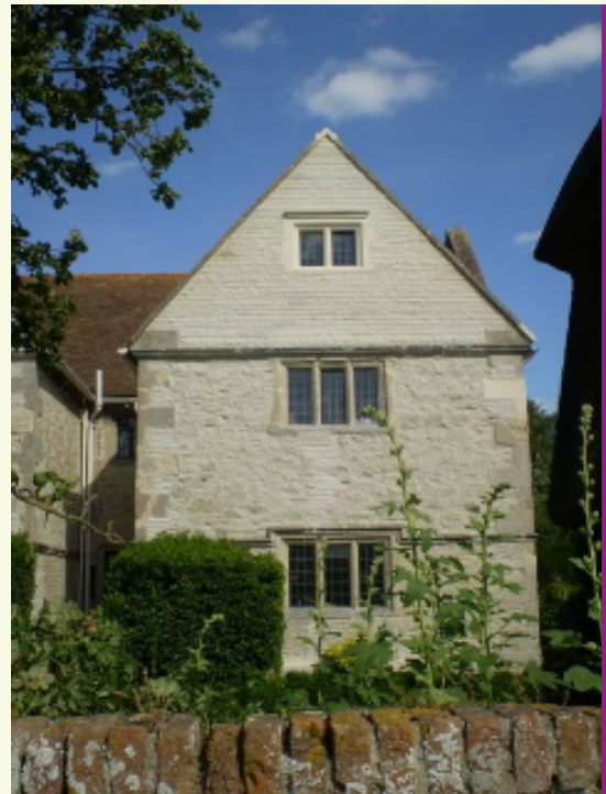
Smalls House, Mackney, showing recent replacement of weathered chalk clunch
